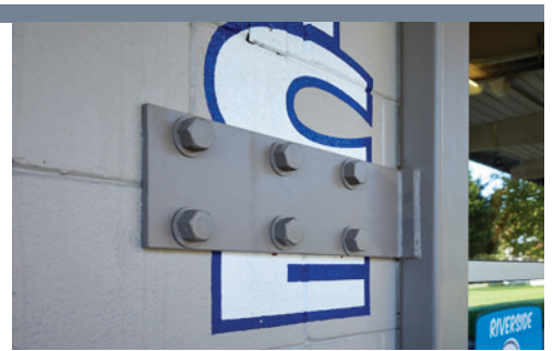
Riverside Elementary School Seismic Retrofit, 2018
