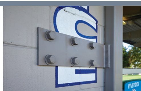
Riverside Elementary School Seismic Retrofit, 2018
