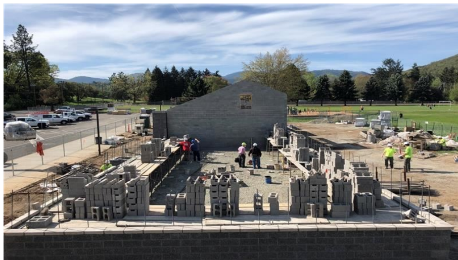
Griffin Creek Elementary School Seismic Rehabilitation and Classroom Addition Medford, Oregon
